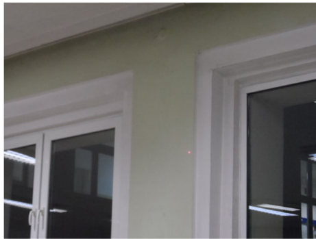
Figure 1. Actual photo of a partition inner surface
